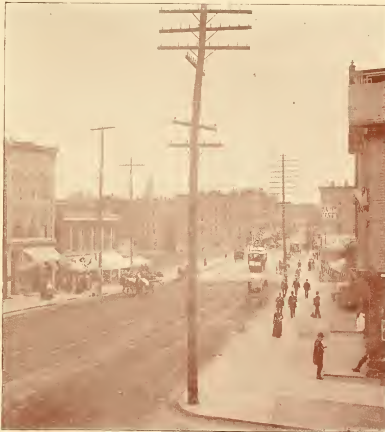
VIEW FROM CORNER OF MAIN AND FRONT STREETS, LOOKING OVER THE BRIDGE TO COURT ST.
